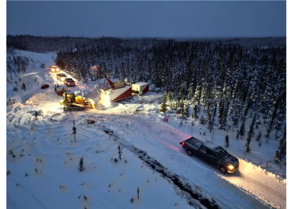
Drill rig on 1 st hole at Douay Porphyry East target (January 2025)
